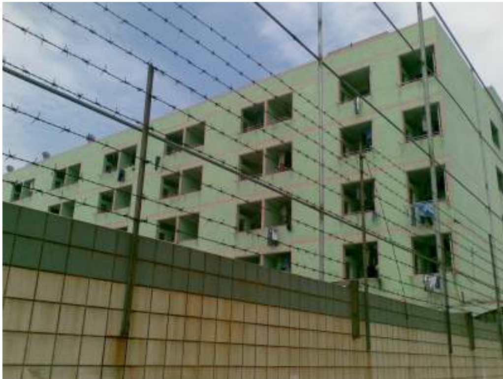
Tianyu worker dormitory.
